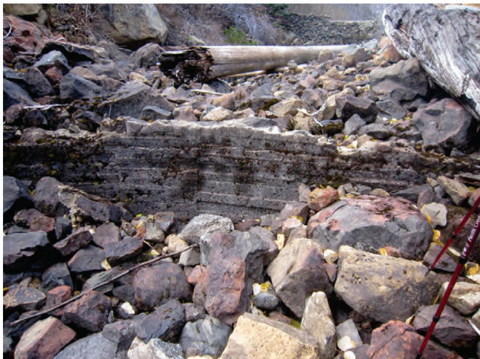
Photograph 12 – Overflow Spillway Channel with Exposed Cutoff Wall
